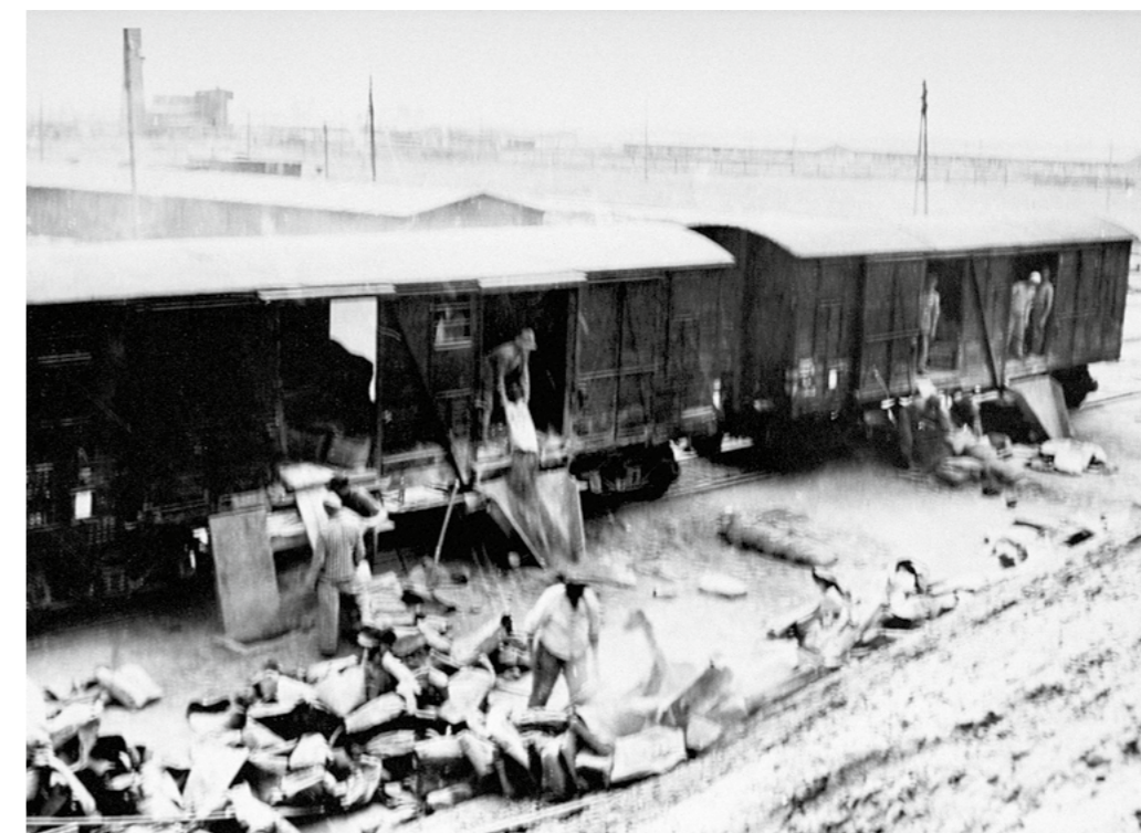
Inmates unload cement sacks from train carriages intended for the construction site of the I.G. Farben factory | Auschwitz, between 1942 and 1945 | Unknown photographer | Washington, D.C., United States Holocaust Memorial Museum
